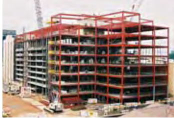
▲ Stage 2 and 5 during construction
