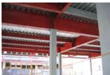
▲ Square hollow section columns support OneSteel primary beams.
