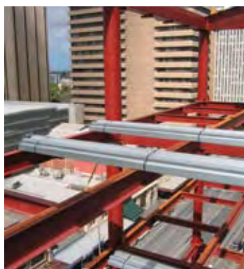
▲ The structural steel decking is predominantly at spans of 2.8 metres.
